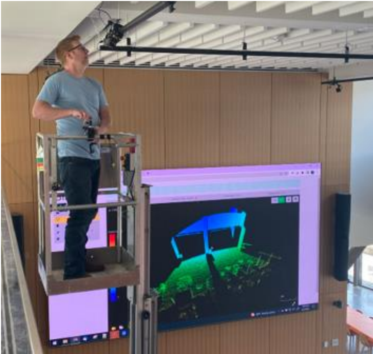
Lidar installation in CID Lobby
